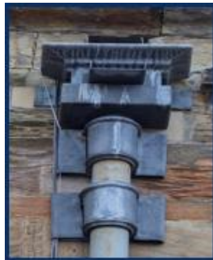
Lead Decorative Embellishments on the Rainwater Pipework at Durham Cathedral
