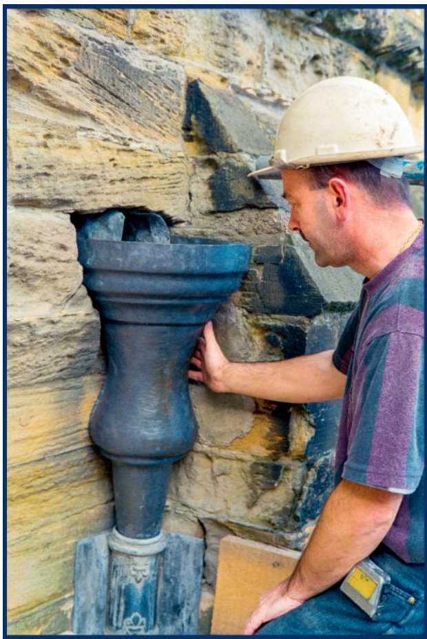
Geoff Kitson Fitting a lead hopper head made in his workshop
